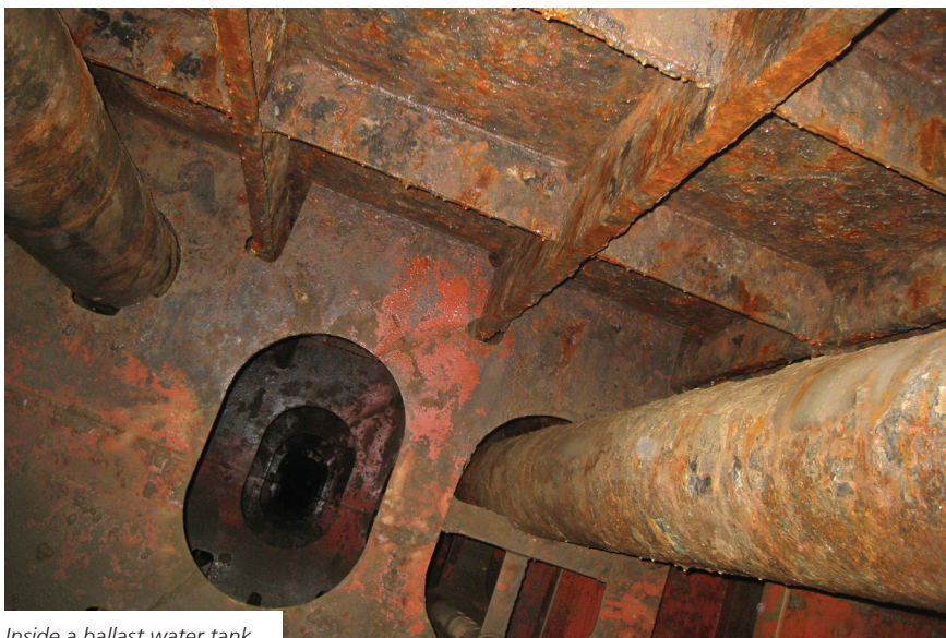
Inside a ballast water tank.
