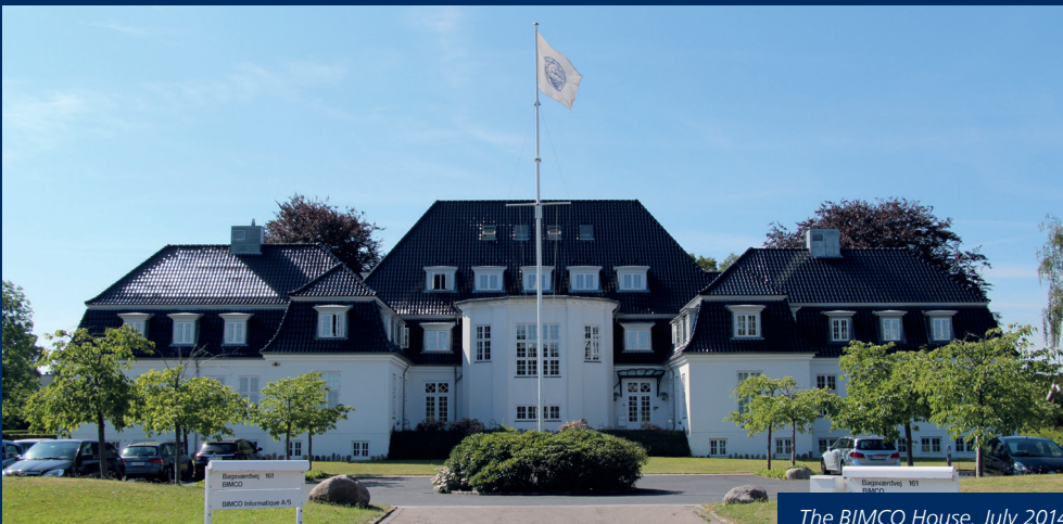
The BIMCO House, July 2014
